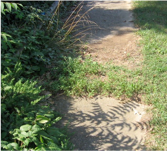
Significant Vegetation on Sidewalk (covering more than half of sidewalk): Photograph by John Evans
