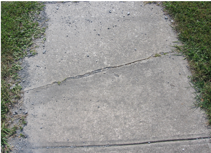
Significant Cracking: Photograph by John Evans
