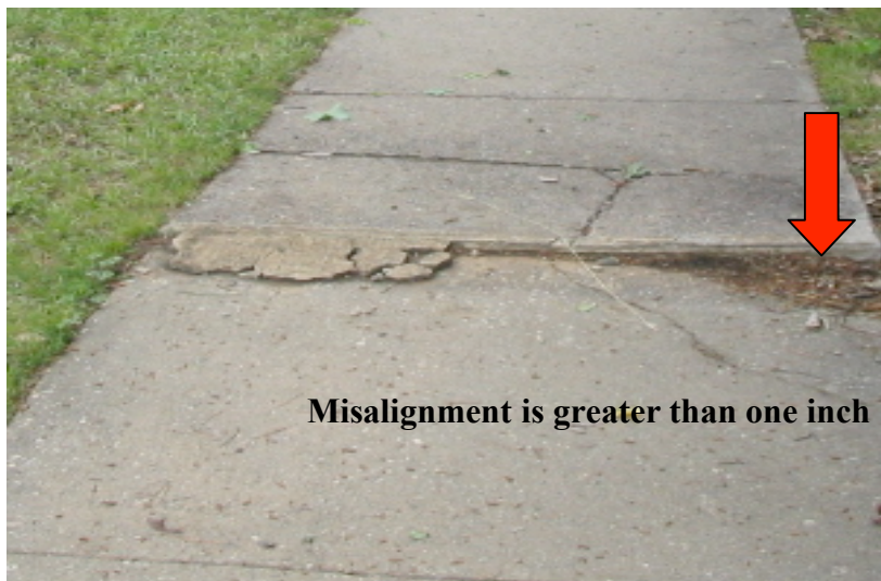
Significant Vertical Displacement: Photo by John Evans
