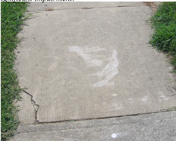
Moderate Surface Deterioration: Photograph by John Evans
