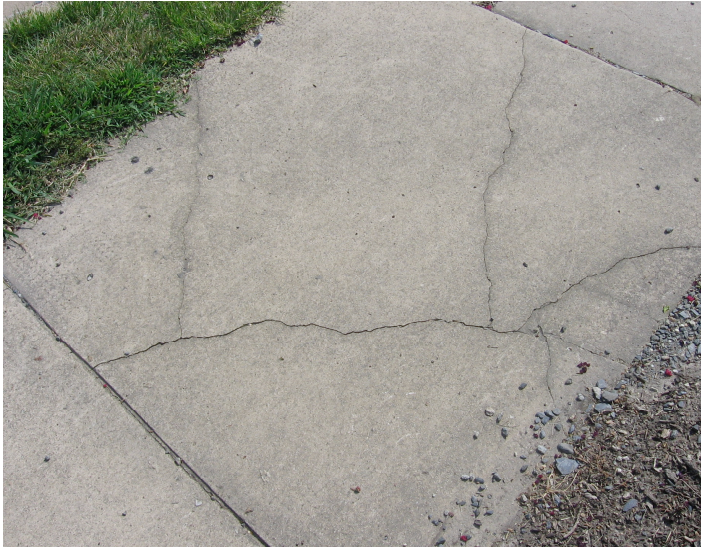
Moderate Cracking: Photograph by John Evans
